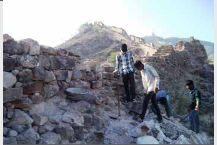
Bhujio Fort restoration work by Karigarshala students
