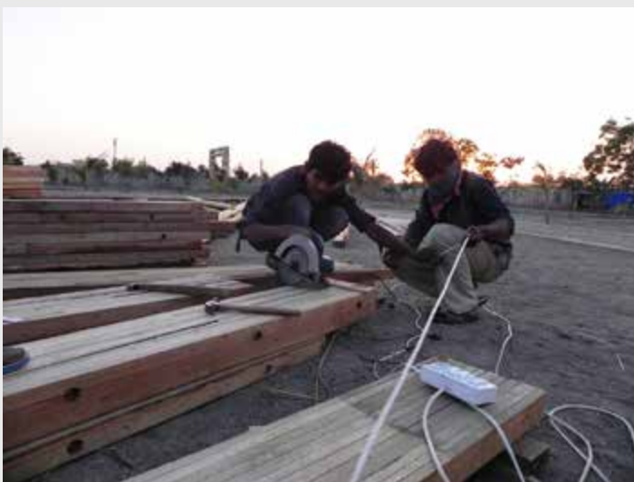
Floorboard construction and installation in progress
