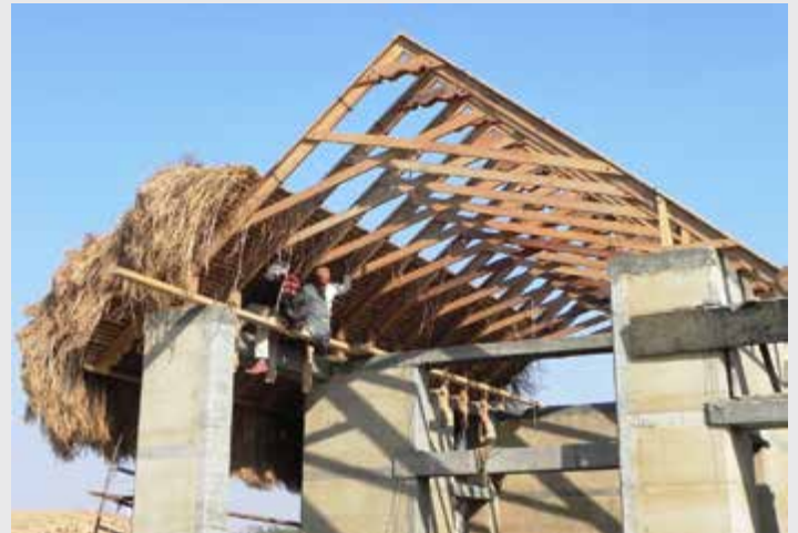
Thatch work in progress at Dr. Vilas Sathey Farmhouse
