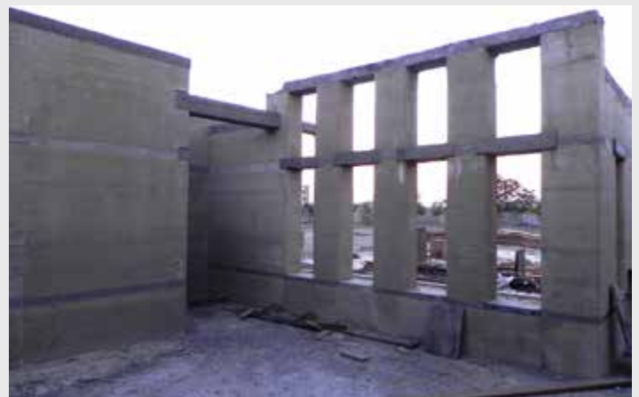
Rammed Earth Walls at Dr. Vilas Sathey Farmhouse
