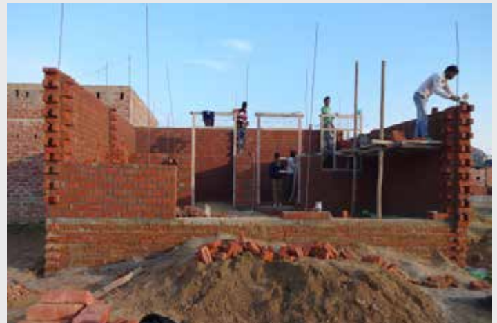
Construction of a house in progress in Shamli
