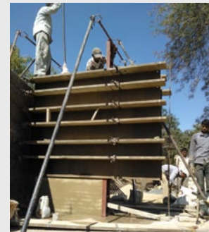
Rammed Earth wall in making
