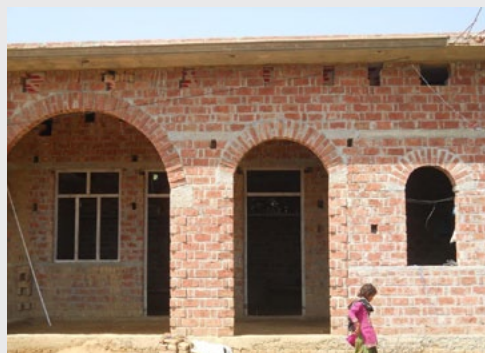
Houses in different stages of construction at Shamli
