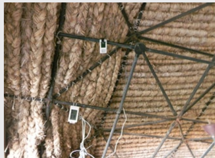
Temperature sensors installed in different roof types
