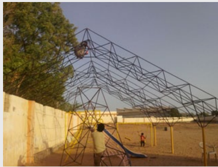
Space frame installed at Sinchan School
