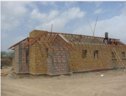
Work in progress for the BMPUS research and office facility
