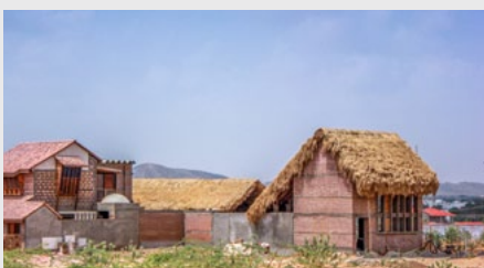
Thatch roof work done by MathaChhaj in Karigarshala
