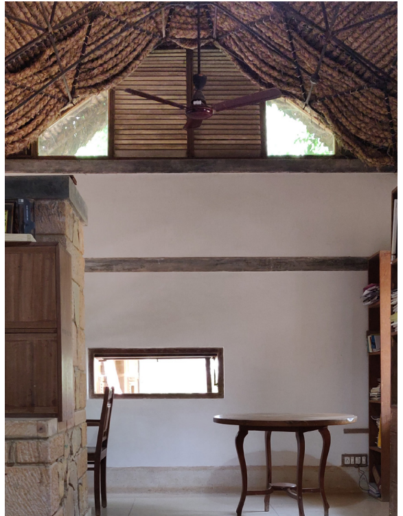
Figure 55. Lime plaster finishes at Jodhpur school and Hunnarshala campus
