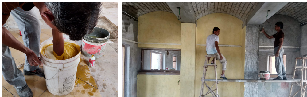
Figure 3. Lime plastering at Jodhpur School
