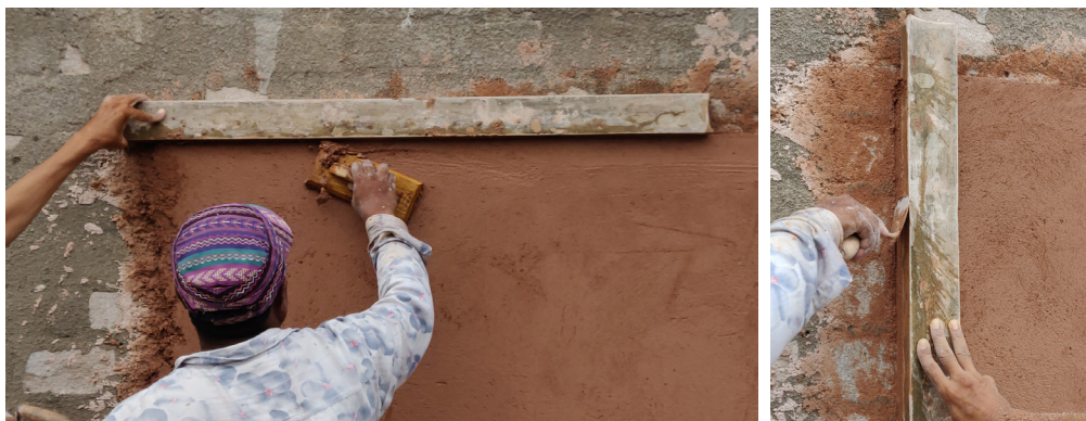
Figure 28. Lime plastering at AINA workshop, Hunnarshala
