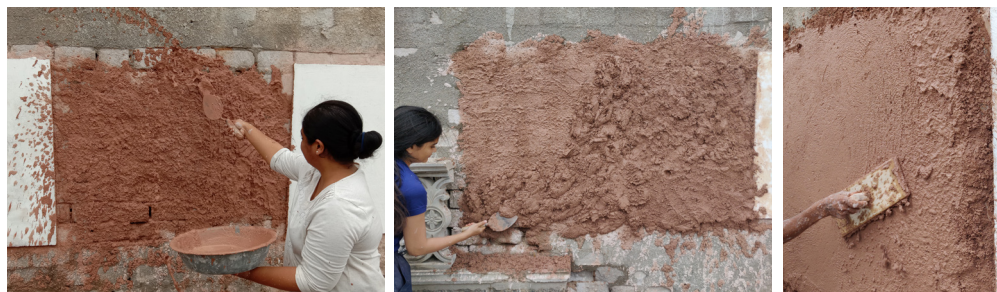
Figure 27. Application of Lime plaster, AINA workshop, Hunnarshala
