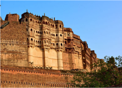
Figure 51. Centuries old forts laid in lime mortar have withstood the tides of time, structural change and climate
