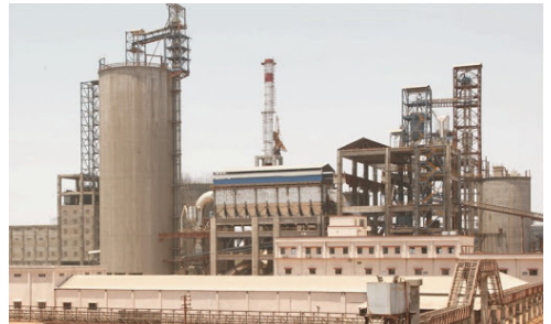
Figure 49. Jaypee cement plant, Gujarat
