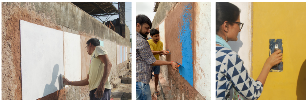
Figure 53. Students at lime plastering AINA workshop at Hunnarshala
