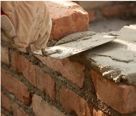
Figure 25. Lime mortar masonry
