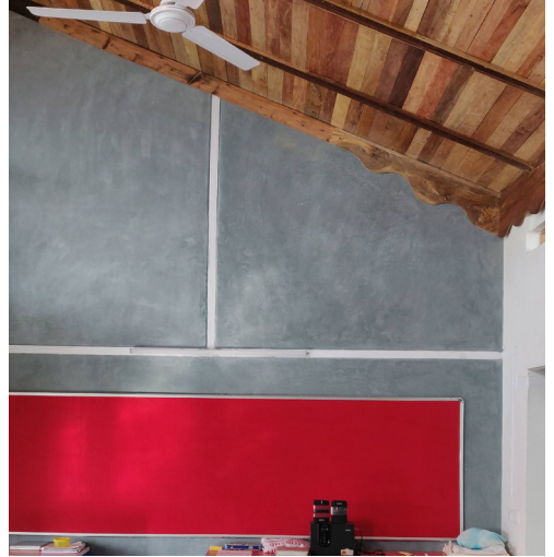
Figure 54. Lime plaster finishes at Jodhpur School
