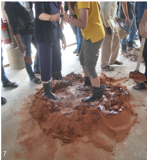
Figure 23. Process of Lime mortar preparation, AINA workshop, Hunnarshala
