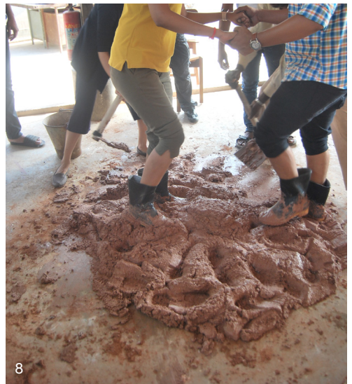
Figure 23. Process of Lime mortar preparation, AINA workshop, Hunnarshala
