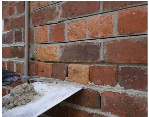
Figure 24. Hydrated lime pointing
