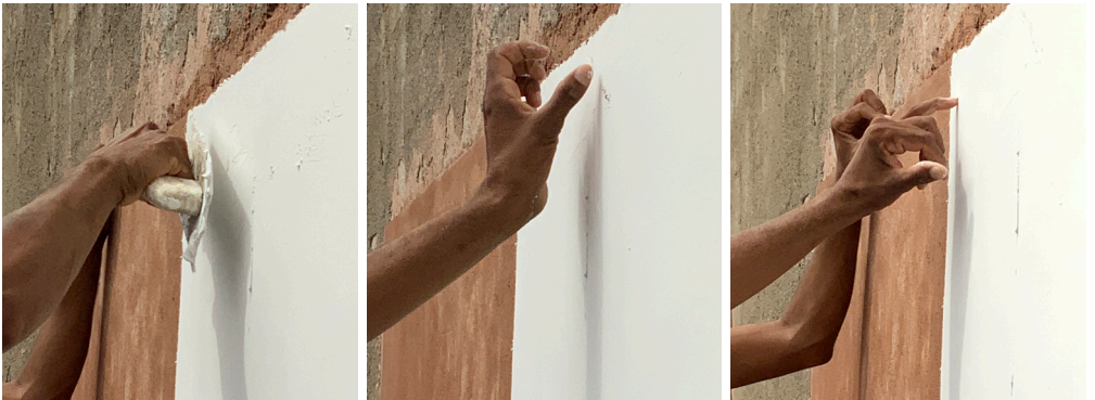
Figure 1. Lime plastering process at AINA workshop (finishing with float and cleaning), Hunnarshala
