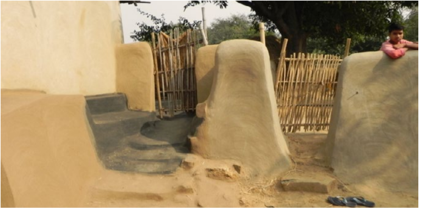
Picture 5: Entrance to a Santhal house, made of earth and finished with different compositions of the same.
