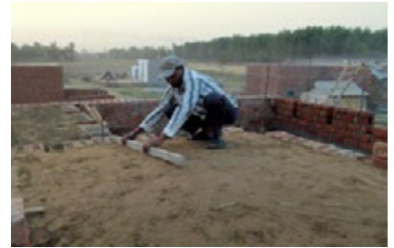
Step 3: Finishing of the form of the dome
