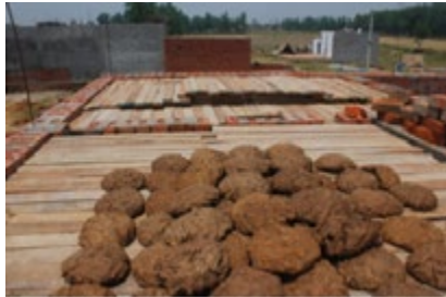
Step 2: Form-work for the shape of dome
