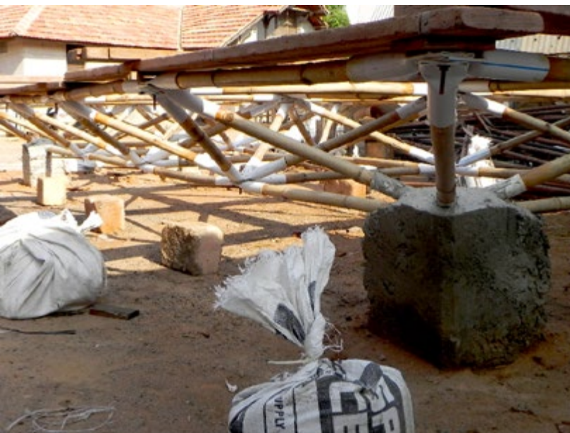
Load testing of spaceframe made out of bamboo
