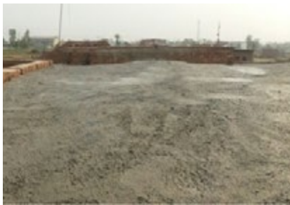
Step 5: Laying of concrete
