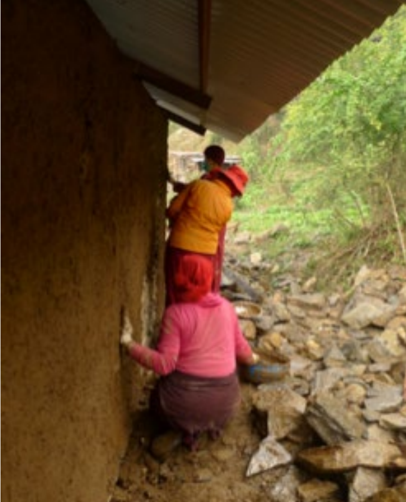
Nuns doing mud plaster on their houses.
