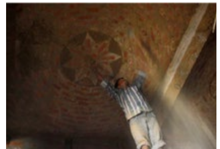
Step 6: Opening of shuttering
