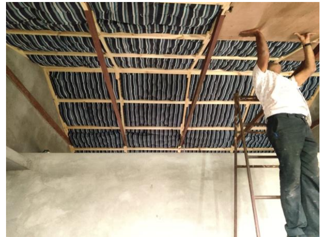
Installing sheep wool insulation panels, Bhuj
