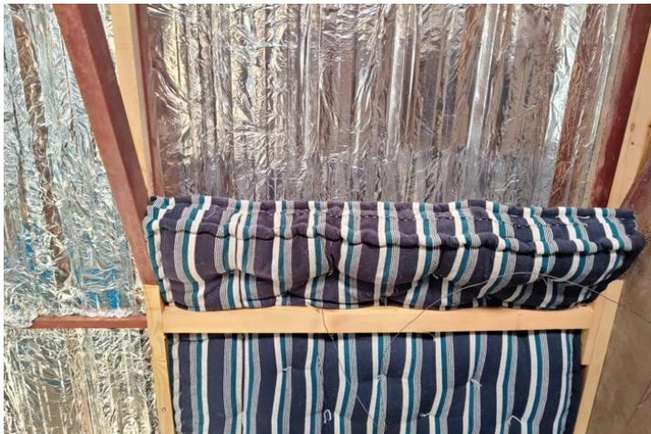
Installing sheep wool insulation panels, Bhuj
