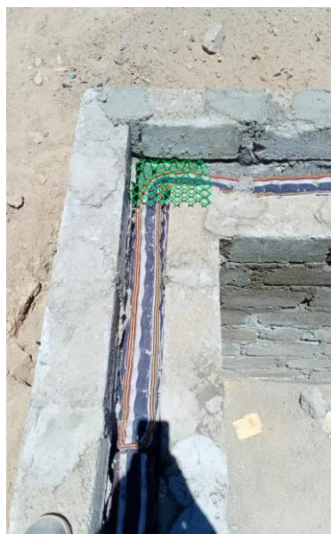
Installing sheep wool insulation panels, Bhuj
