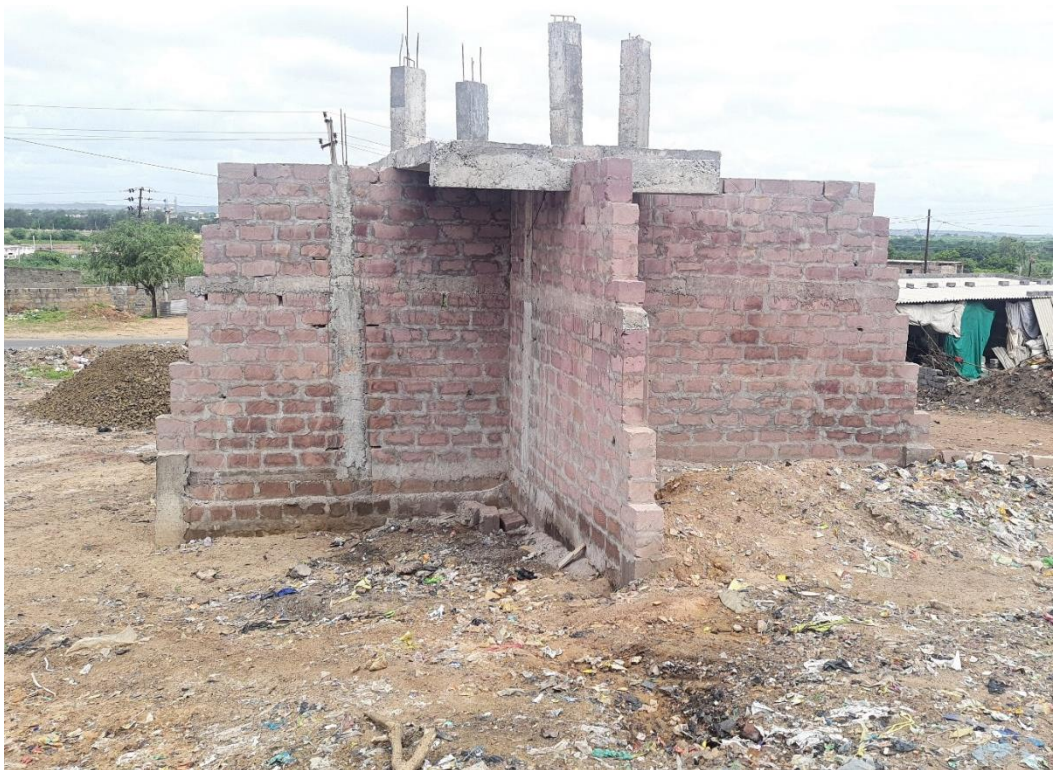
Vibrator Screening Completed Civil Work
