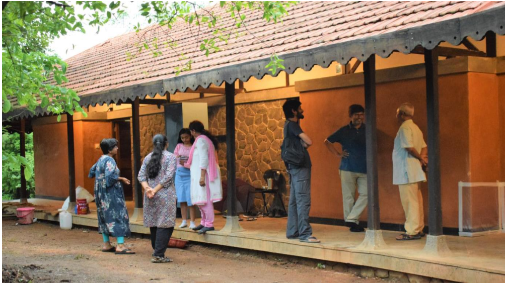
Guest House Block-2 completed & inaugurated at Sahyadri School
