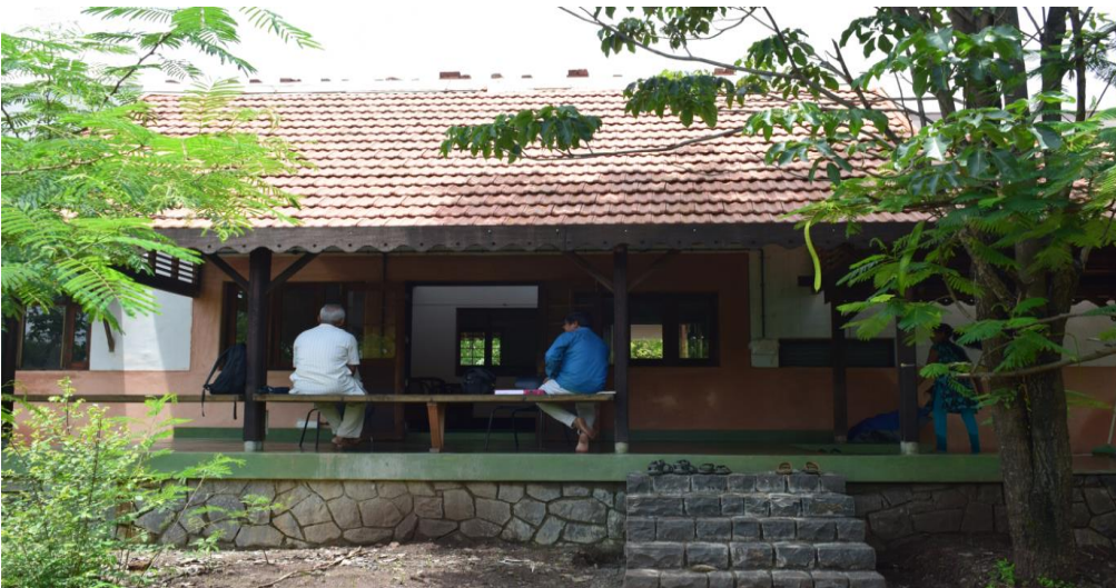
New Admin building completed & inaugurated at Sahyadri School
