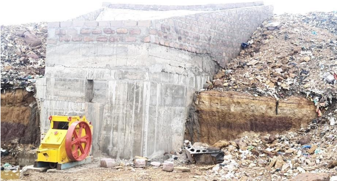
Crusher Machine and Hopper
