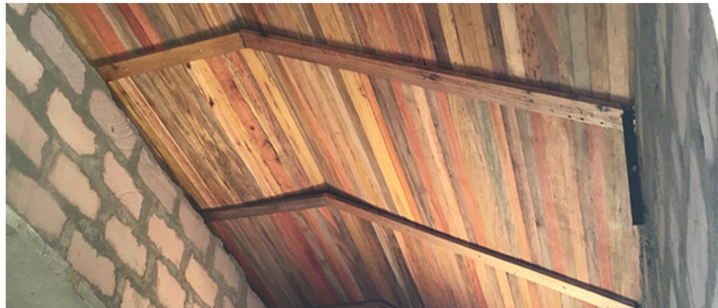
1. Mangalore tile with woden planks
