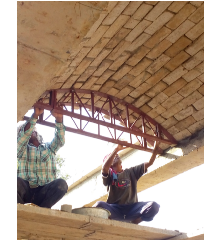
VAULTS IN PROCESS WITH STABILIZED ADOBE
