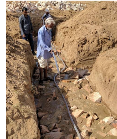
SAND - PACKED FOUNDATION
