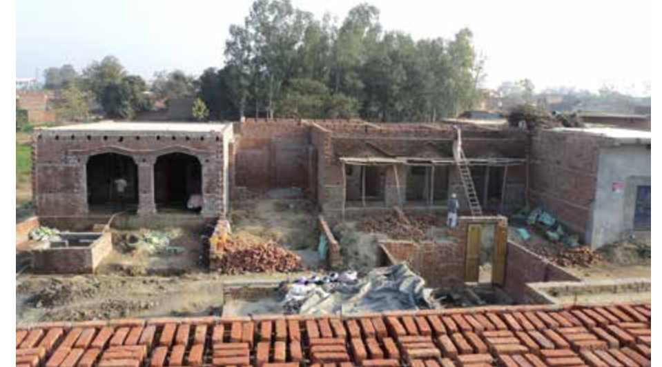
A house construction in Bassikalan
