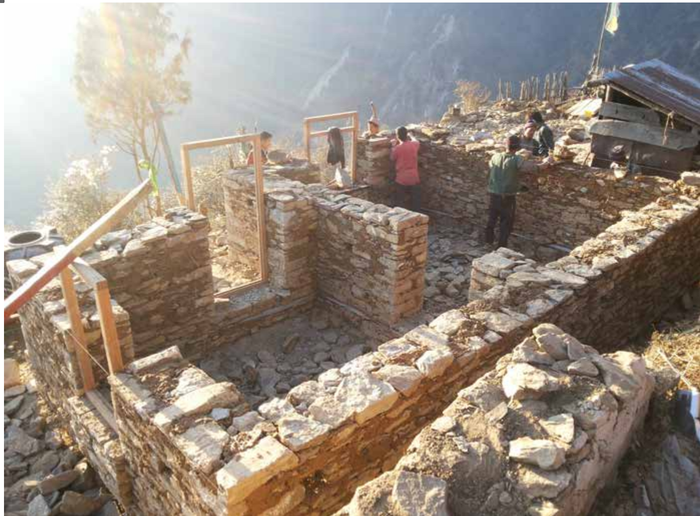
The houses for nuns under construction
